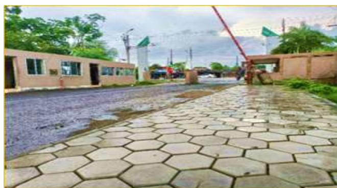
Picture 2.0: Laid Pavement Blocks at CLC Gate-03
