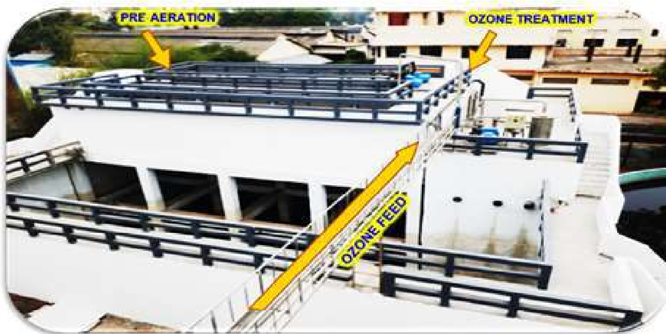
Fig.4 : Ozonation System - Pre-Aeration & Ozone Reaction Chamber and Treated Effluent Storage Tank
