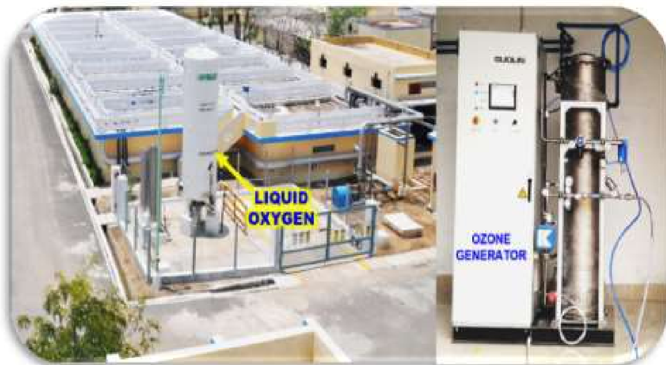
Fig.2 : Ozone treatment is found more effective and safer for application than liquid oxygen
